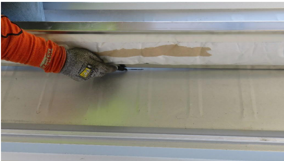
Marking inside of curb
