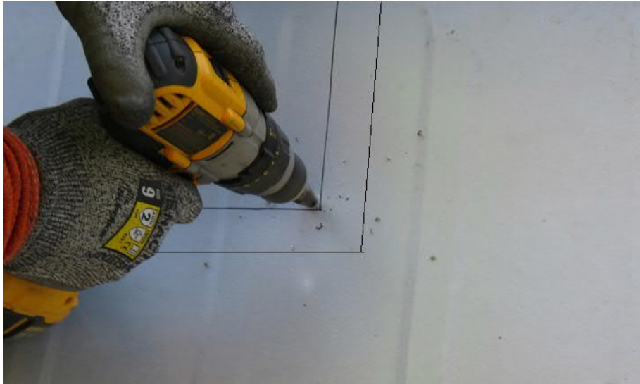
Drill Corners of cutout.
